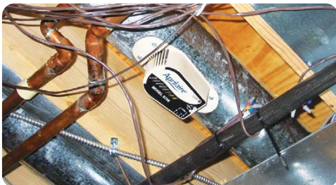
Imagine trying to install a "shell" type damper here!
